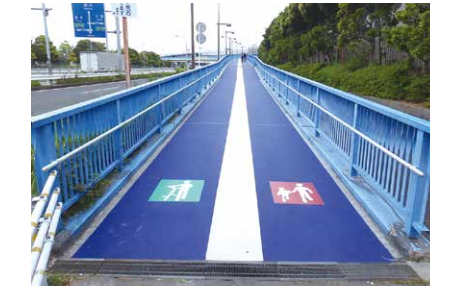
Bicycle pedestrian road maintenance
